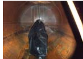
Bladder Installed Through Tank Opening (View From Inside Tank)
