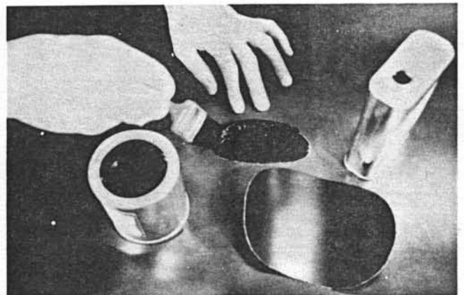
8-01-5. Clean both the roughened area and the patches with specified solvent.
